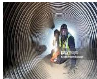
Fig 1. Confined Space Entry.
